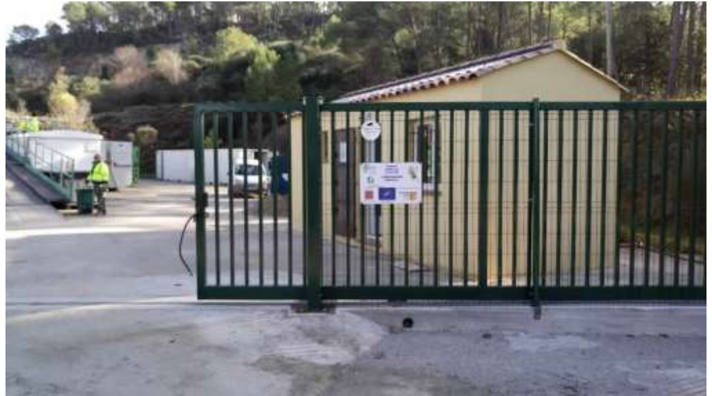
View of the entrance after the renovation operation
